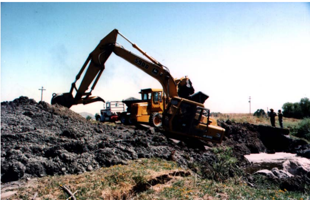
Pile of excavated material grows as infiltration gallery is constructed
