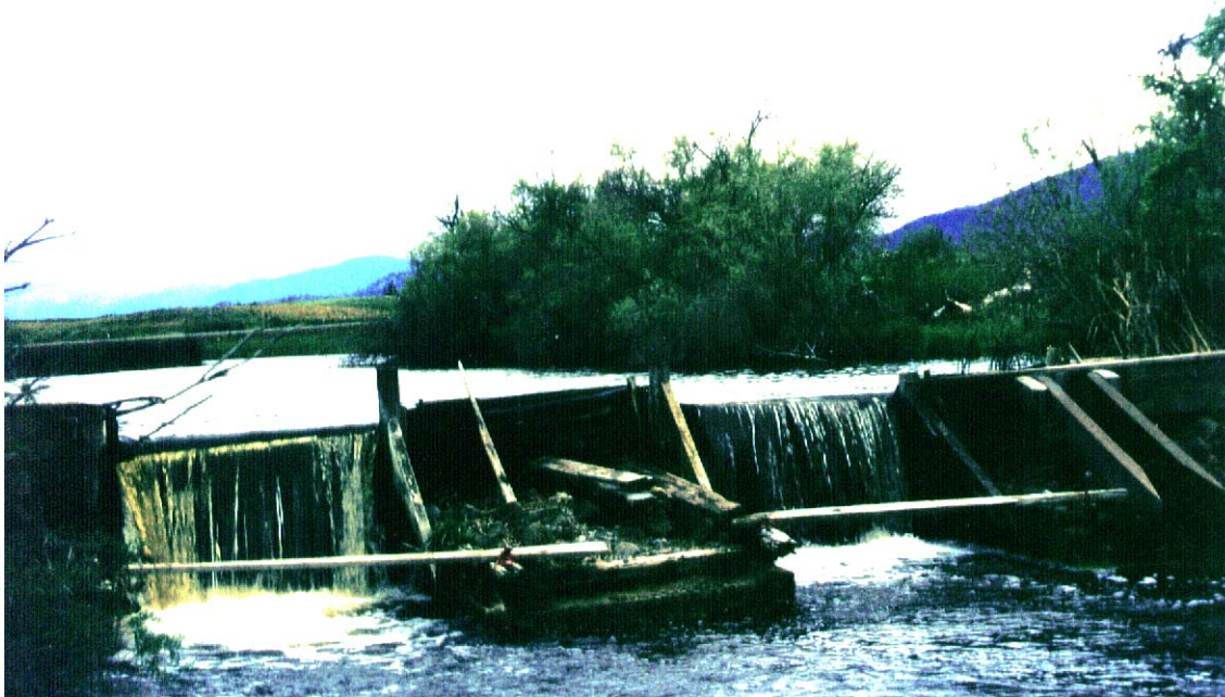
Fiock dam, summer, 1992
