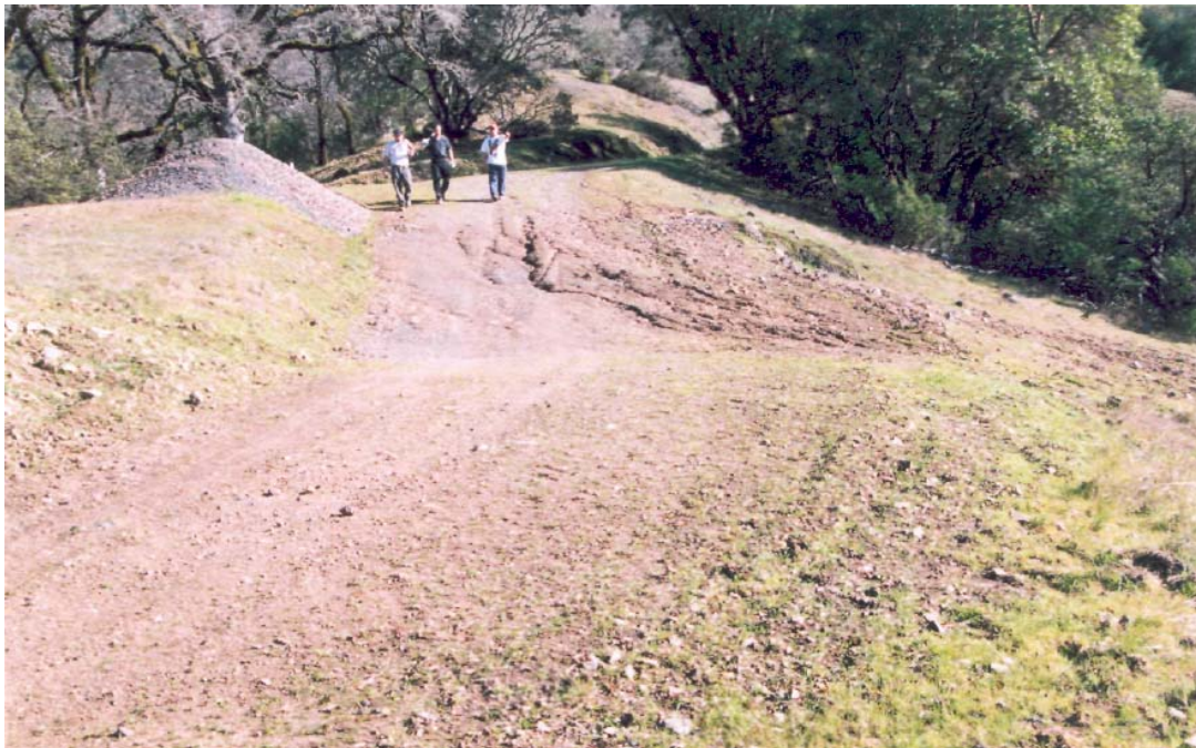
Figure 11. The erodability of the soil and the spacing between rolling dips dictates the extent of erosion occurring on the road bed. This rolling dip shows rills developing on the road bed when the road grade steepens, however all the sediment is deposited on the hillslope beyond the road with no sediment delivery to nearby streams.
