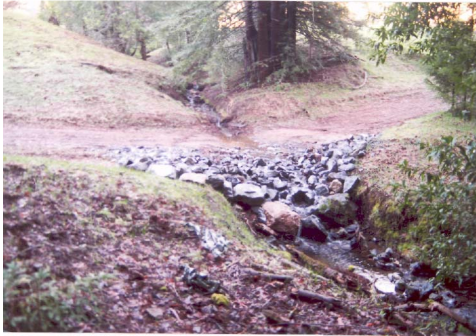
Figure 8C. View upstream at Site #44 one winter after installation. The stream must flow over the armored apron at all stream flows to function properly and prevent future sediment delivery to stream channels.
