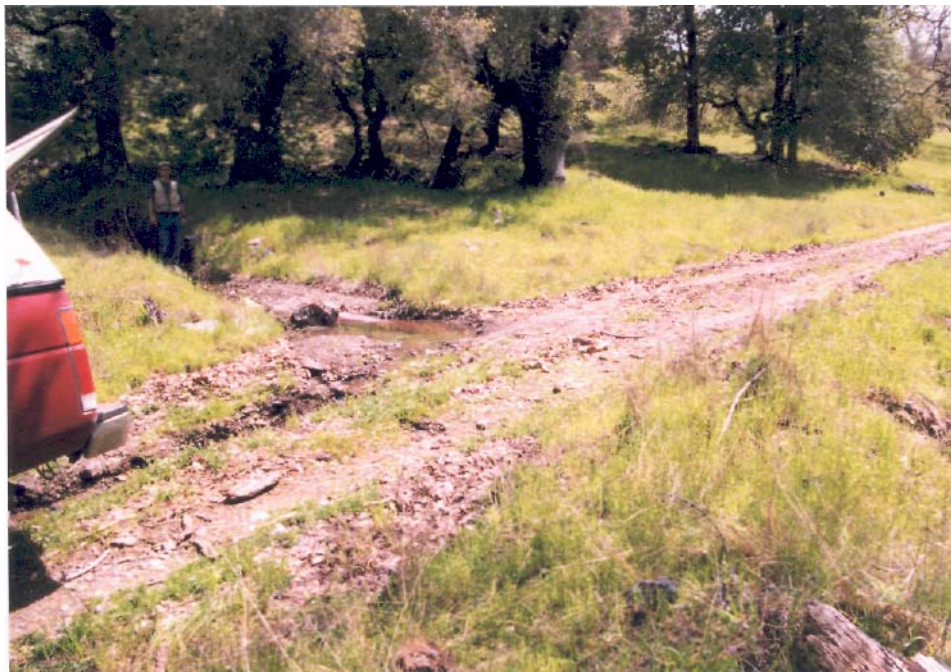
Figure 1A and 1B. Examples of typical erosional problems in Austin Creek State Recreation Area which lead the State Parks and PWA to seek CDF&G funding to protect important aquatic habitat in the East Austin Creek watershed. Failed stream crossings and direct sediment delivery (upper photo), un-culverted diverted streams resulting in hillslope gully erosion and sediment delivery (lower photo).
