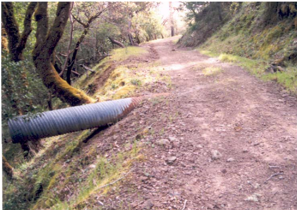
Figure 2A and 2B. Examples of typical erosional problems in Austin Creek State Recreation Area which lead the State Parks and PWA to seek CDF&G funding to protect important aquatic habitat in the East Austin Creek watershed. Large road bed drainage areas between ditch relief culverts resulting in the formation of large man-made channels (hillslope gullies) and direct sediment delivery (upper photo), long lengths of un-controlled or un-planned road drainage resulting in high sediment delivery rates of road bed. surface lowering erosional products (lower photo).
