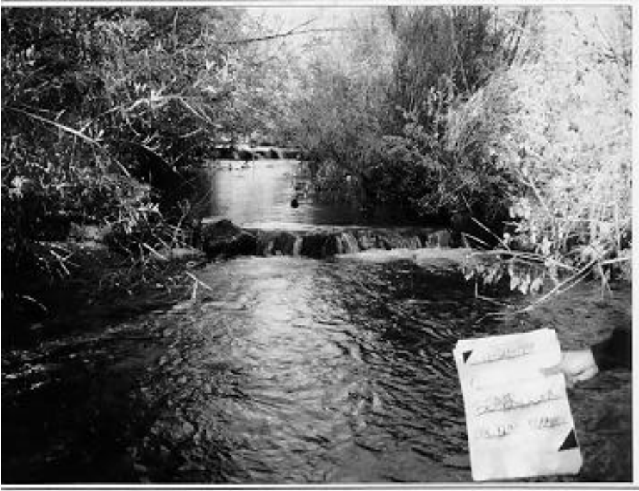
Figure A5-15. Boulder weirs in lower Beaver Creek in fall 1994. Notice encroaching riparian. Photo courtesy Klamath National Forest.
