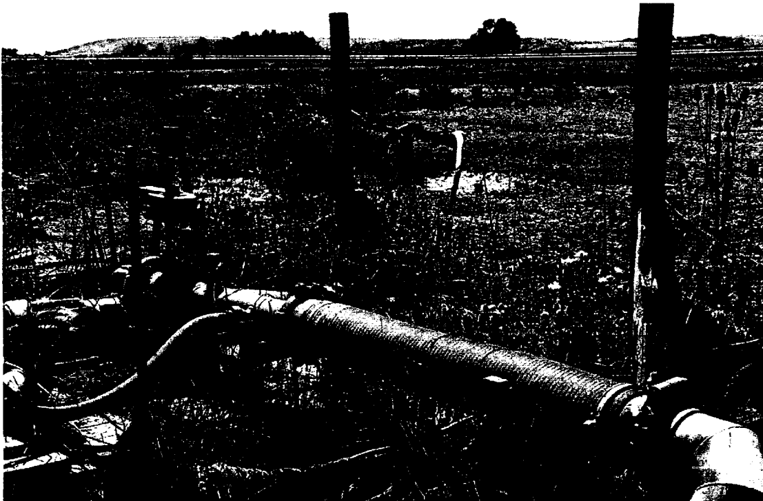
Figure A5-37. Pump installed at Fiock Ranch to eliminate the need for a diversion dam on the lower Shasta River. Dam removal should help improve dissolved oxygen conditions locally.
