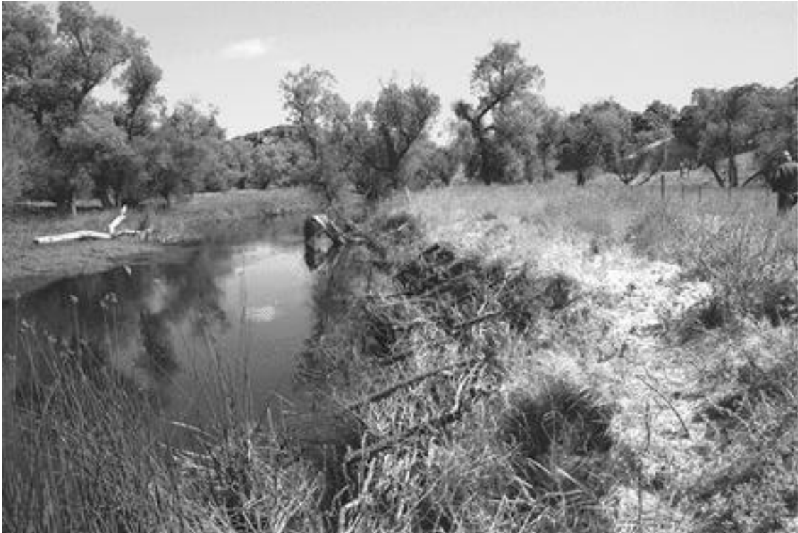
Figure A5-43. Willow waddles used for bank stabilization at the Easton Ranch along the Shasta River during project construction. Photo courtesy Dave Webb.
