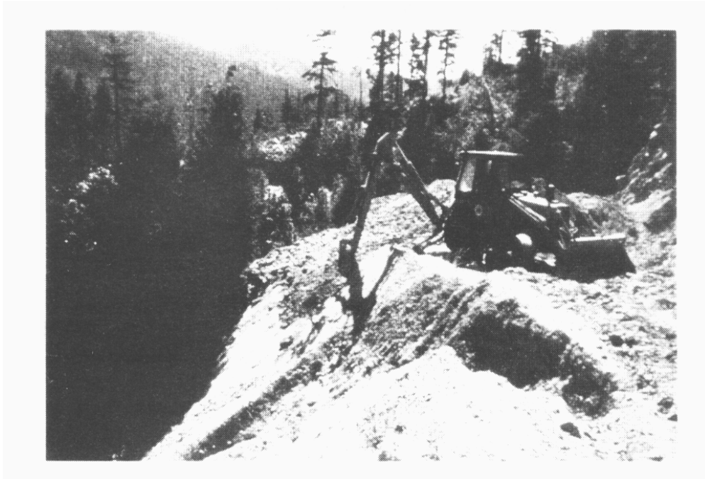
Figure 3-6 -- Putting roads "to bed" in Hoopa Reservation watersheds has reduced erosion and helped streams to recover.
