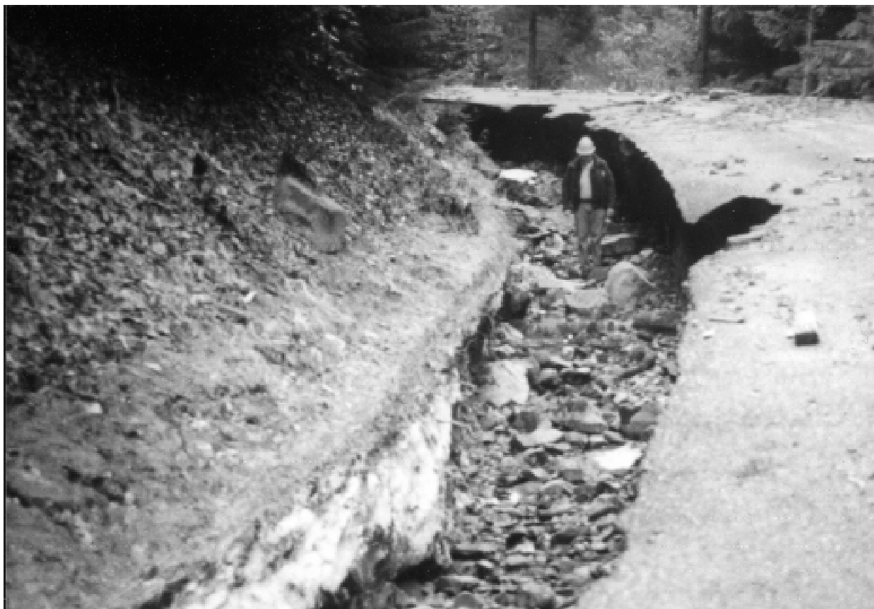
Figure 10—Diversion of streamflows at stream crossings can have large erosional consequences far removed from the initial failure site. Here water diverted along the inboard ditch for several hundred meters initiated additional crossing failures along the way. Photo courtesy of the Siskiyou National Forest.
