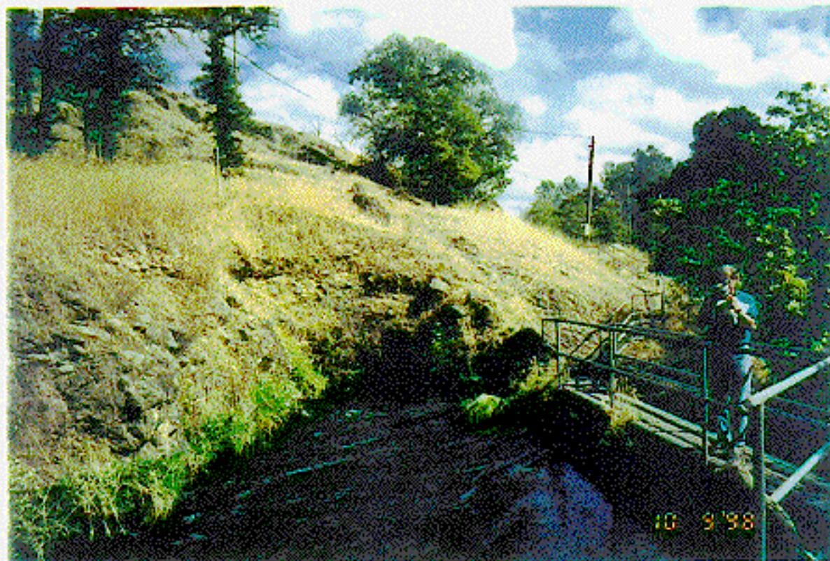
Photograph 11. - Inskip Canal tunnel outlet portal (footbridge shown over wasteway).
