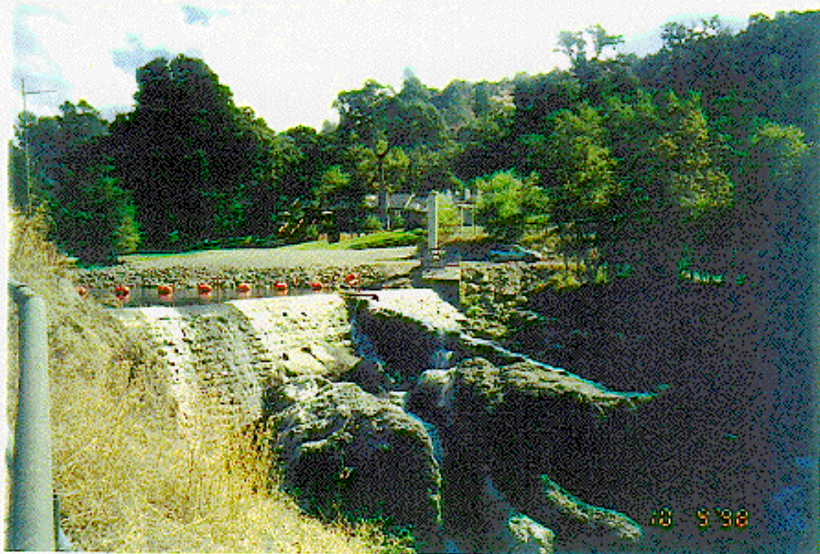
Photograph 10. - Downstream face of Inskip Diversion Dam.
