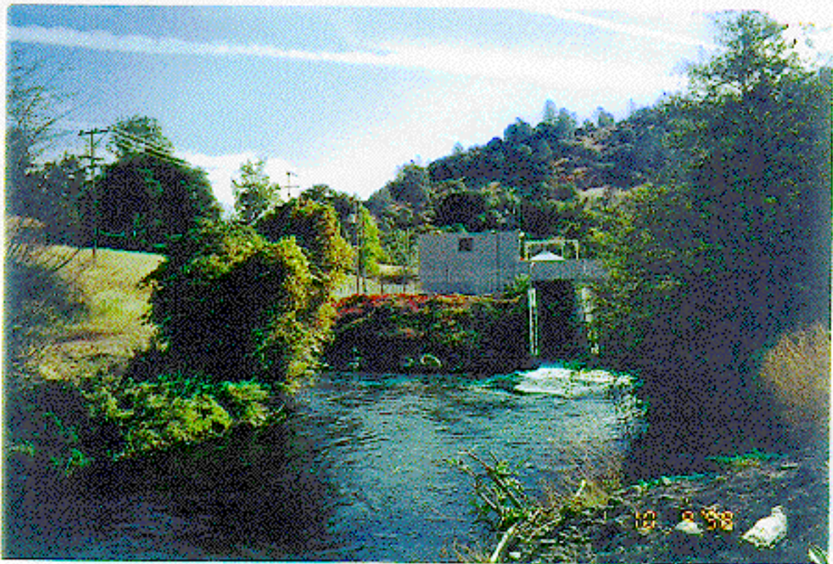
Photograph 2. - South Powerhouse and tailrace channel, looking upstream.
