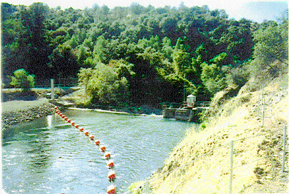
Photograph 7. - Upstream view of Inskip Diversion Dam (canal headworks at right).
